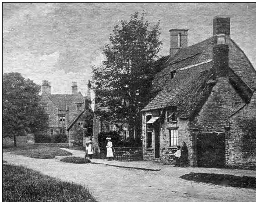
1 Main Street, 1904 [Jack Hart collection] Home of Frederick Skillington, now the community village shop
