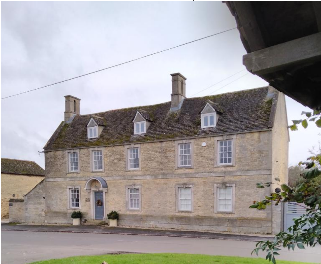
Manor House, Main Road, [next to Black Bull, opposite Church]
